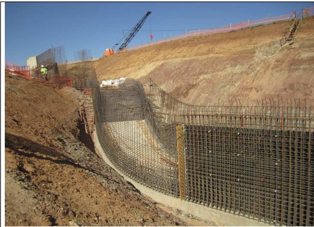
Tailrace channel discharging onto the existing stilling basin of Botterkloof Dam
