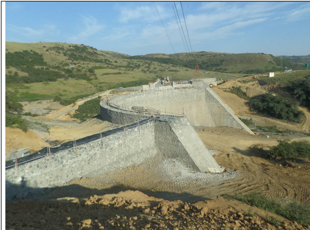
Photo of Mndwaka Dam nearing completion taken from the Cable Way
