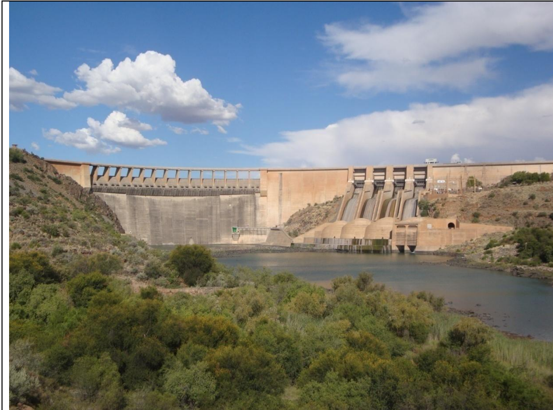
Van der Kloof Dam in the Orange River
