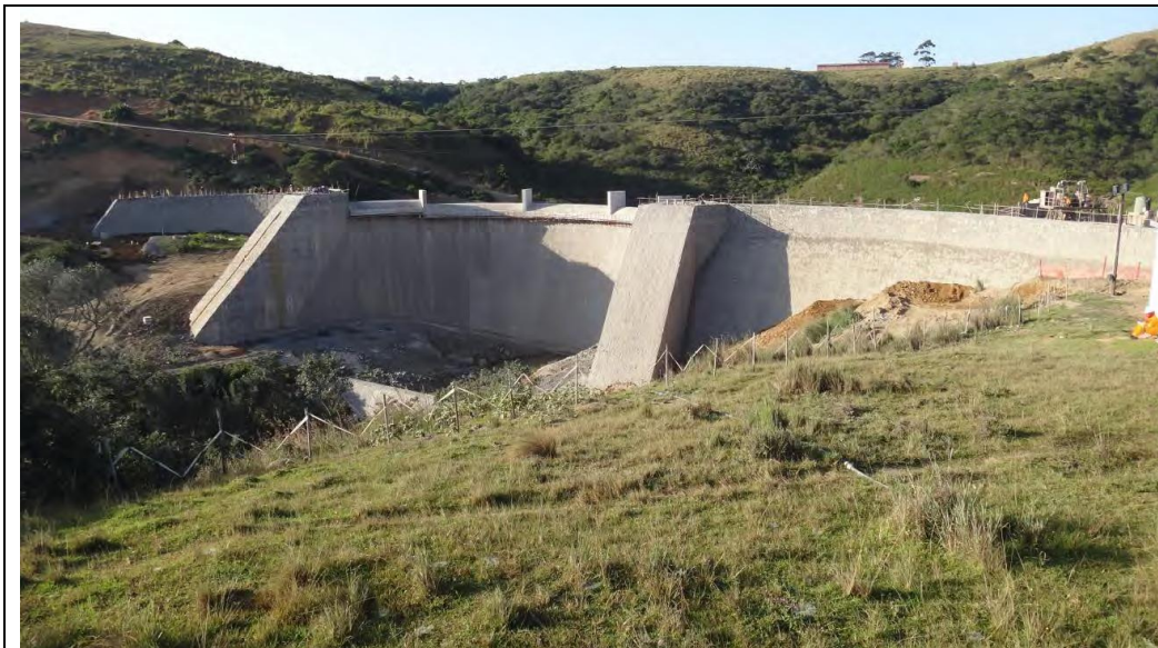
Photo of Mndwaka Dam nearing completion taken from the left flank
