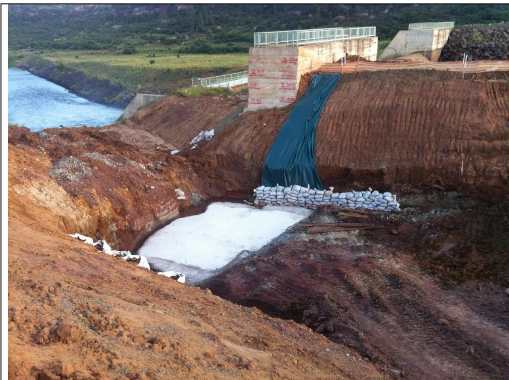
Casting of blinding concrete onto intake works foundation
