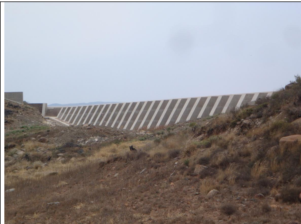
Grassridge Dam near Middelburg in the Eastern Cape
