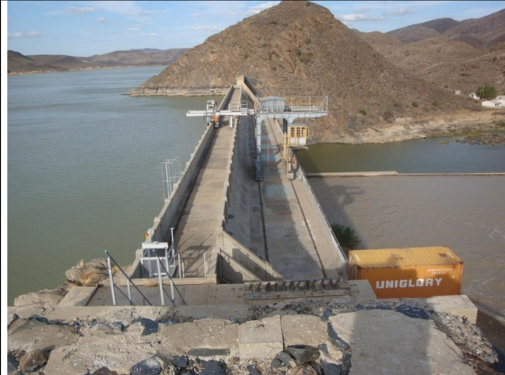
Floriskraal Dam near Laingsburg in the Western Cape
